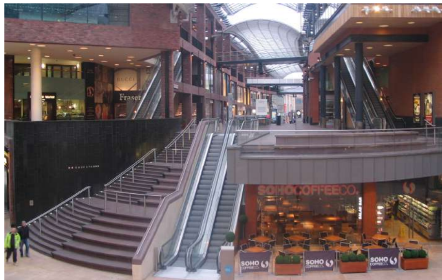
House of Fraser Shopping Mall, England
